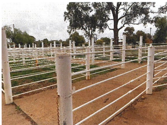
Photo 1: Metal structure white paint throughout, refer sample WSP-131150 - positive for lead paint
